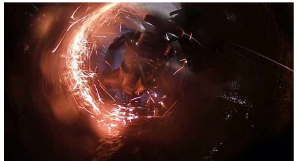
CUTTING A CAST IRON TAP
