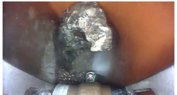
UHP CONCRETE REMOVAL
