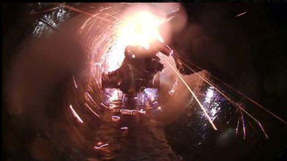
CUTTING A CAST IRON TAP
